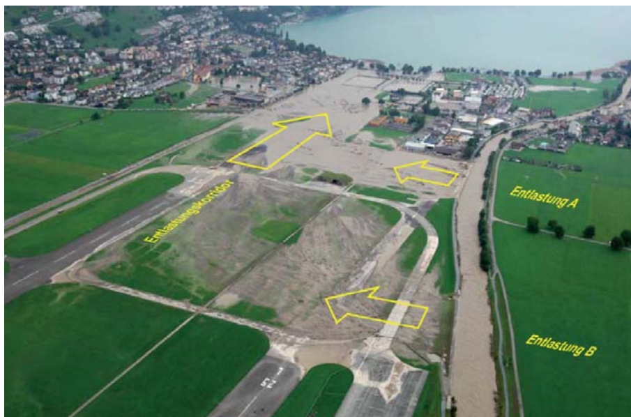
Figure 14: Example of the Engelberger Aa: the excess water leaves the river channel and flows through the discharge corridor towards Lake Lucerne.
